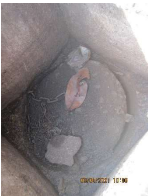
IMG_1440.jpg – Underneath the steel plate covering the restrooms wastewater collection system.
