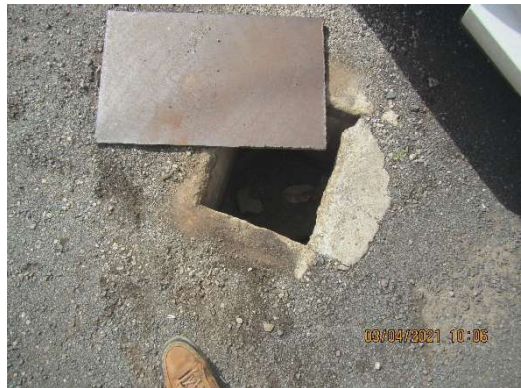
IMG_1439.jpg – Steel plate covering wastewater collection system for the two restrooms.
