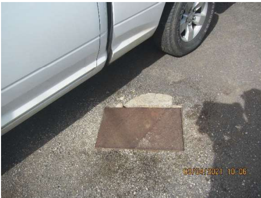
IMG_1438.jpg – Steel plate covering wastewater collection system for the two restrooms.
