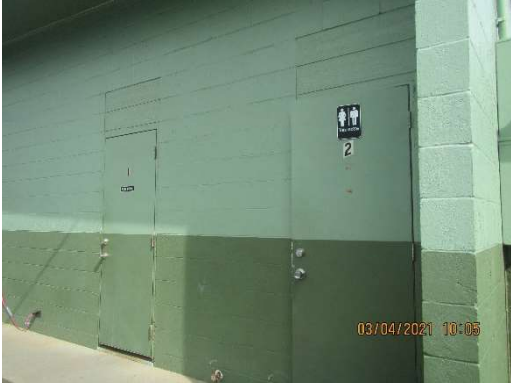
IMG_1436.jpg- Overview of the two restrooms located on the west side of the former service station building.
